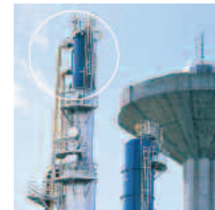
Direct mounting of a spiral condenser at a stripper tower reduces installation costs, increases product recovery and reduces pollutant escape.
